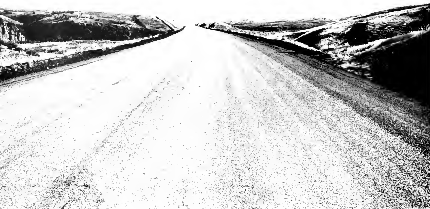
View looking south over section of highway built by State from point a half mile south of Poso Creek
